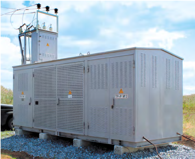
High voltage MDS in transportation position
